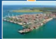
Colon Container Terminal
